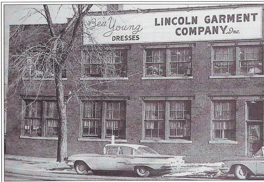
The factory building built by the Lincoln Commercial Club, at 220-226 N. Chicago Street. Lincoln, Illinois: A Pictorial History.
